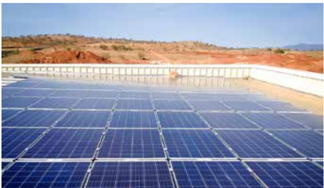
ROOF-SOLAR BITUME / 151,7 kWc Maroc
